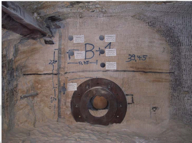
Figure 5.4 Photograph of the BAMBUS II re-excavation.
